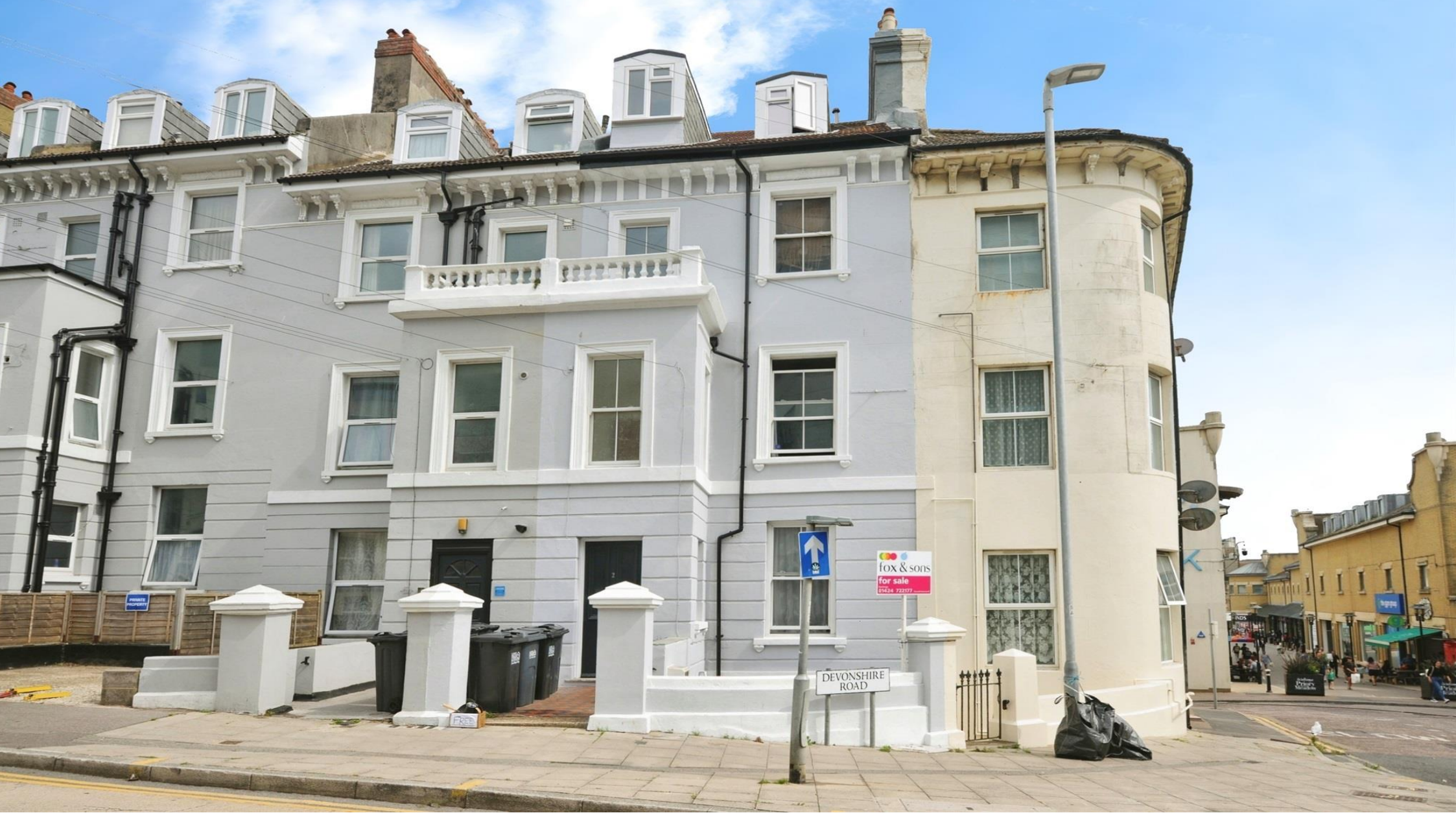
Flat 1 Devonshire Road, Hastings TN34 1NE
