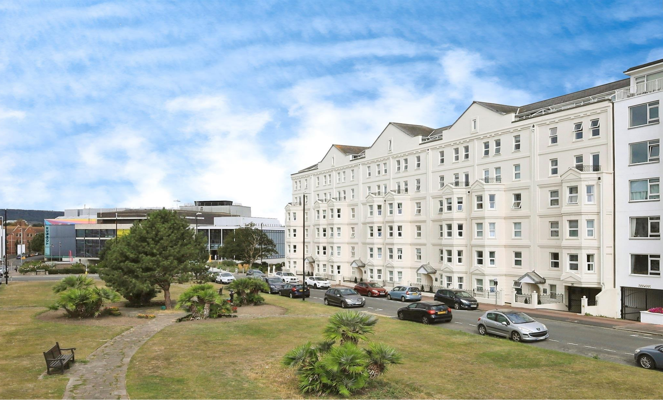
Berkeley Court Wilmington Square, Eastbourne BN21 4DX
