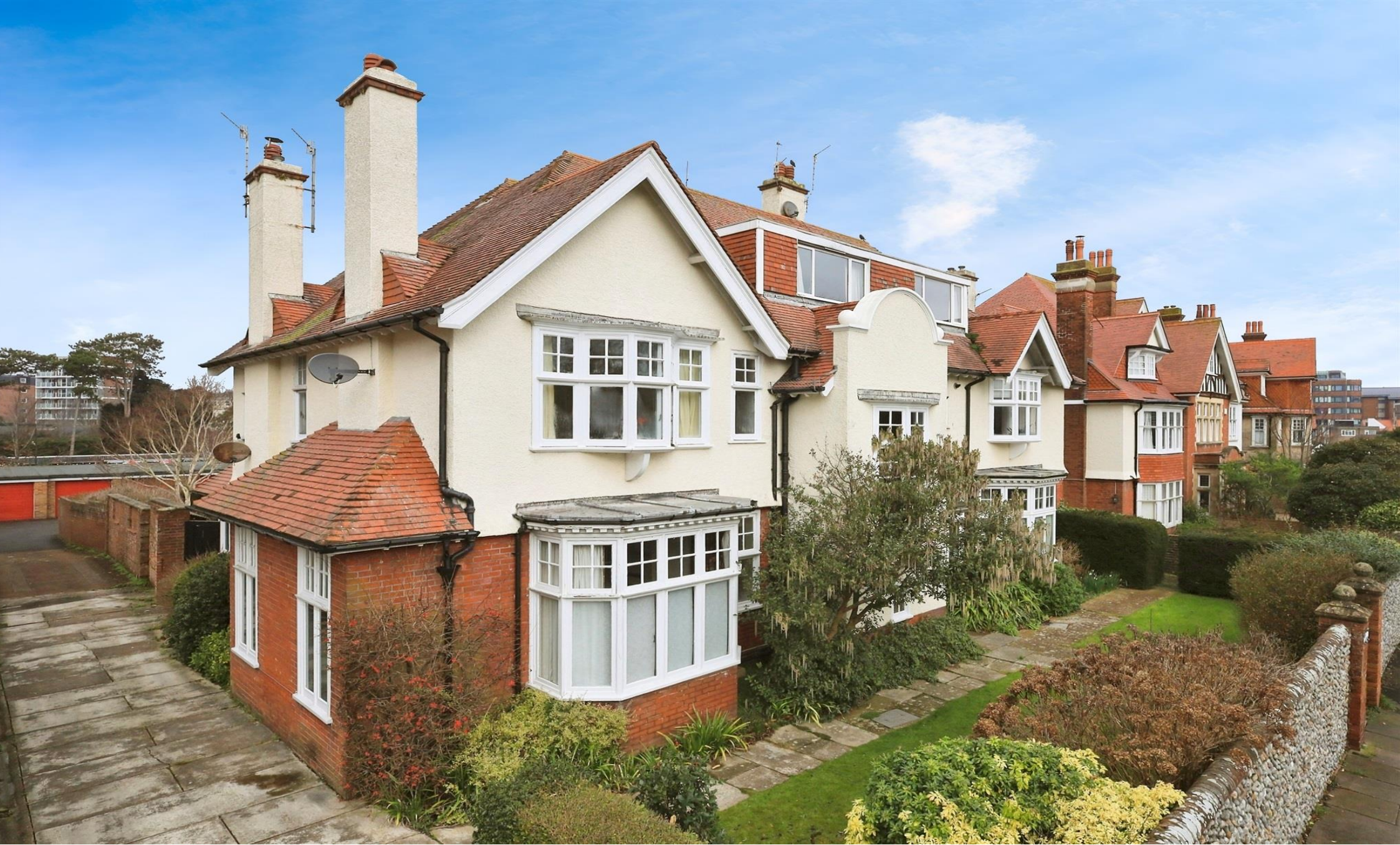
Aymond Grange Dittons Road, Eastbourne BN21 1DW
