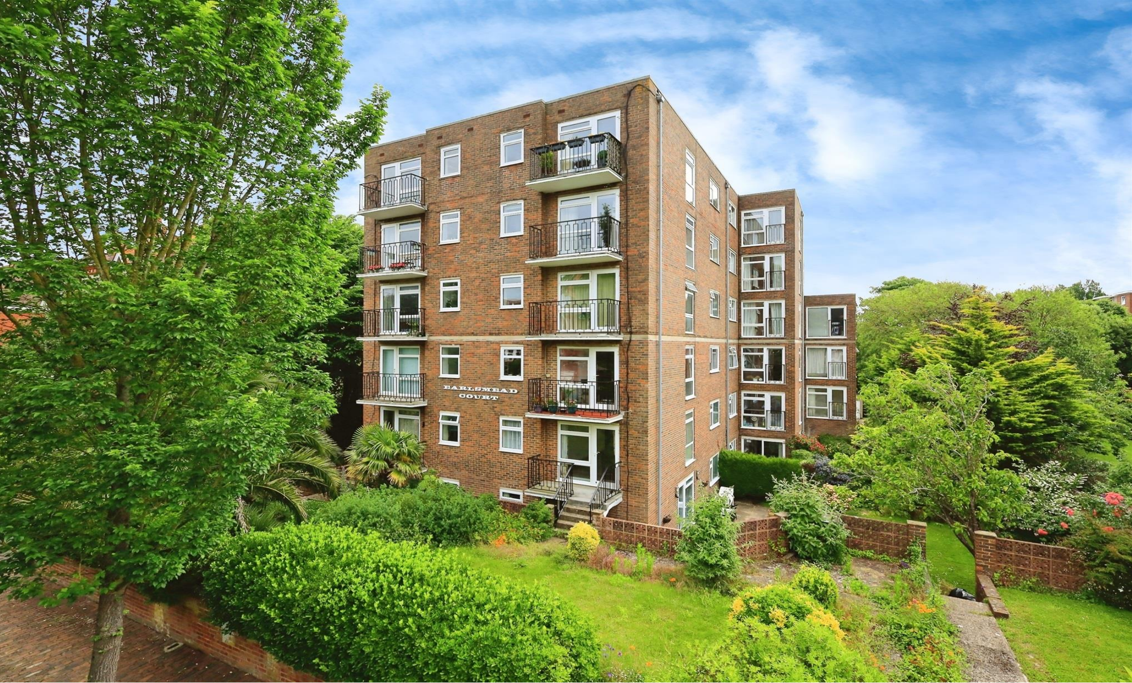
Earlsmead Court Granville Road, Eastbourne BN20 7HE
