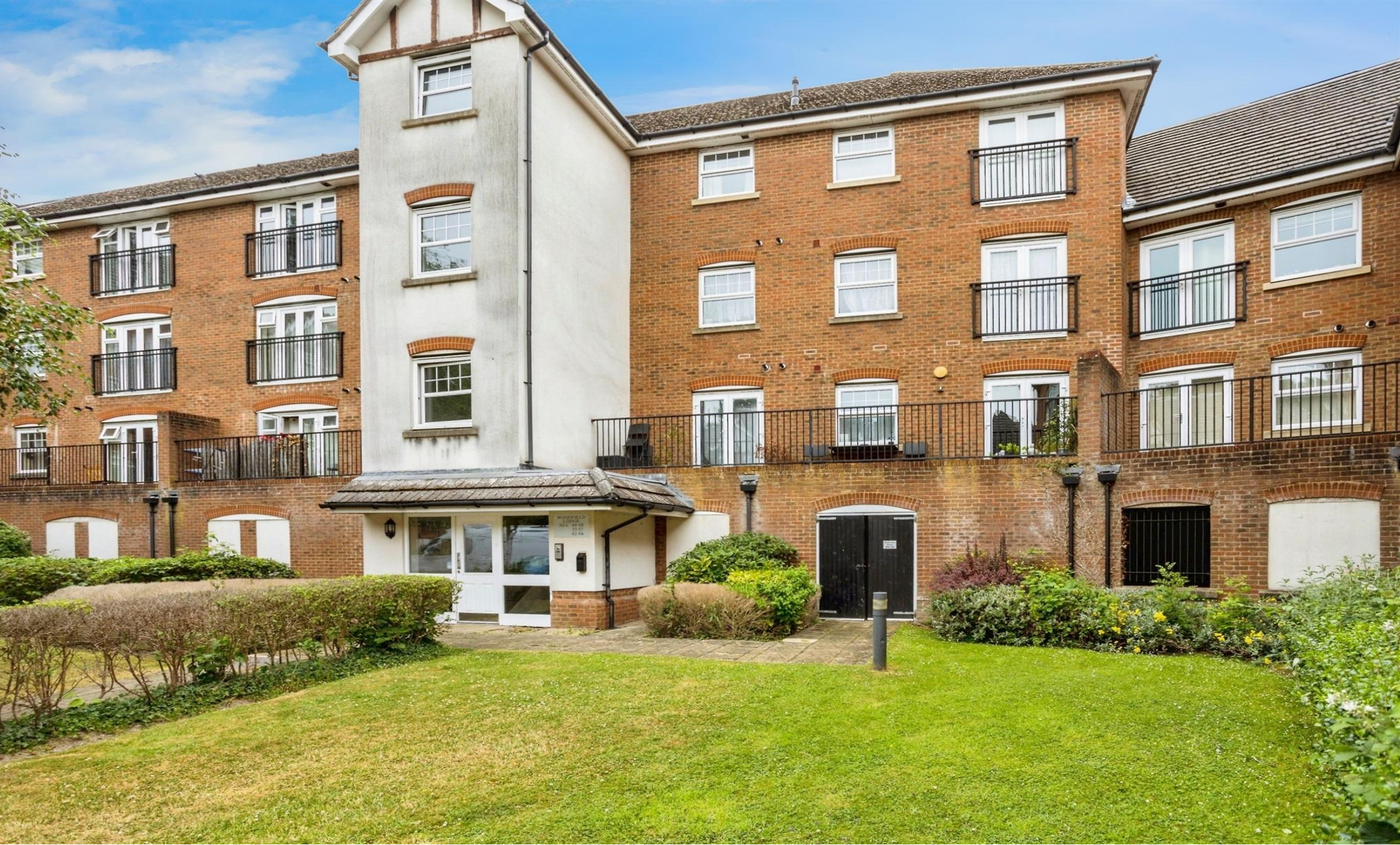
Woodfield Lodge, Woodfield Road, Crawley, RH10 8AH
