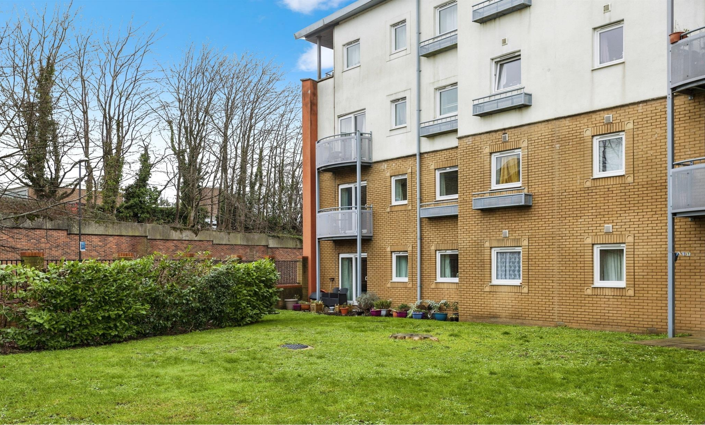
Reeves House Trafalgar Gardens, Crawley RH10 7SW
