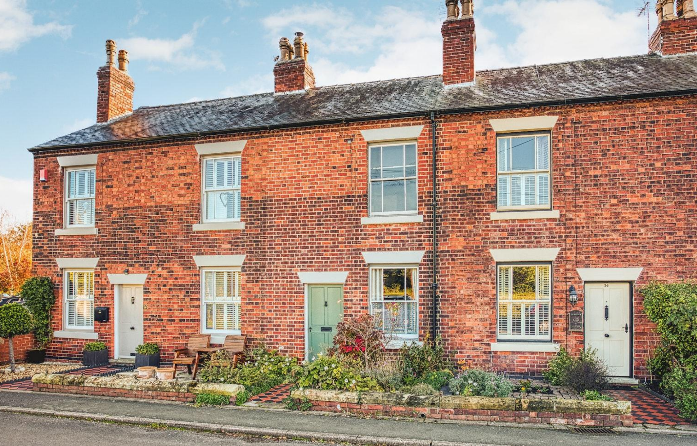
The Wharf, Shardlow, Derby
