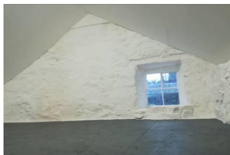
Boiler room loft
