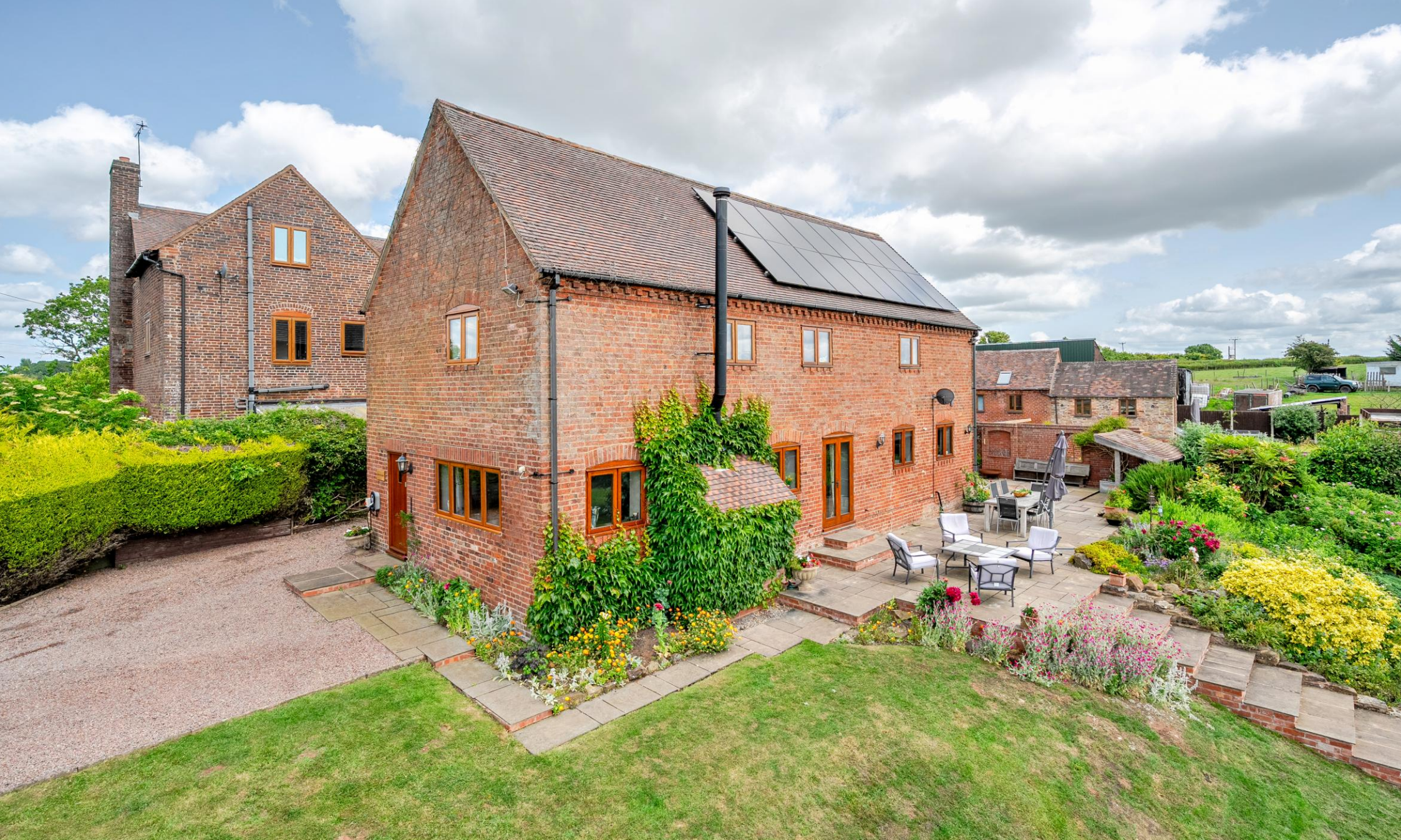
Oakwood Barn, Heightington
