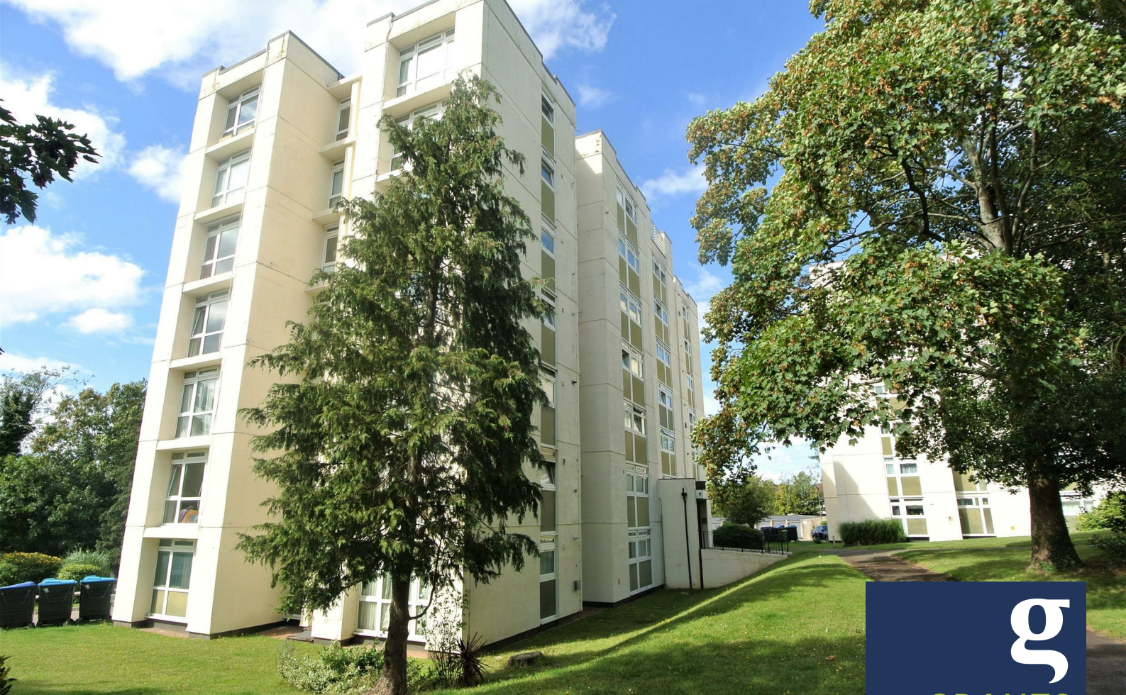
Manor Court, Weybridge, KT13 8RF
