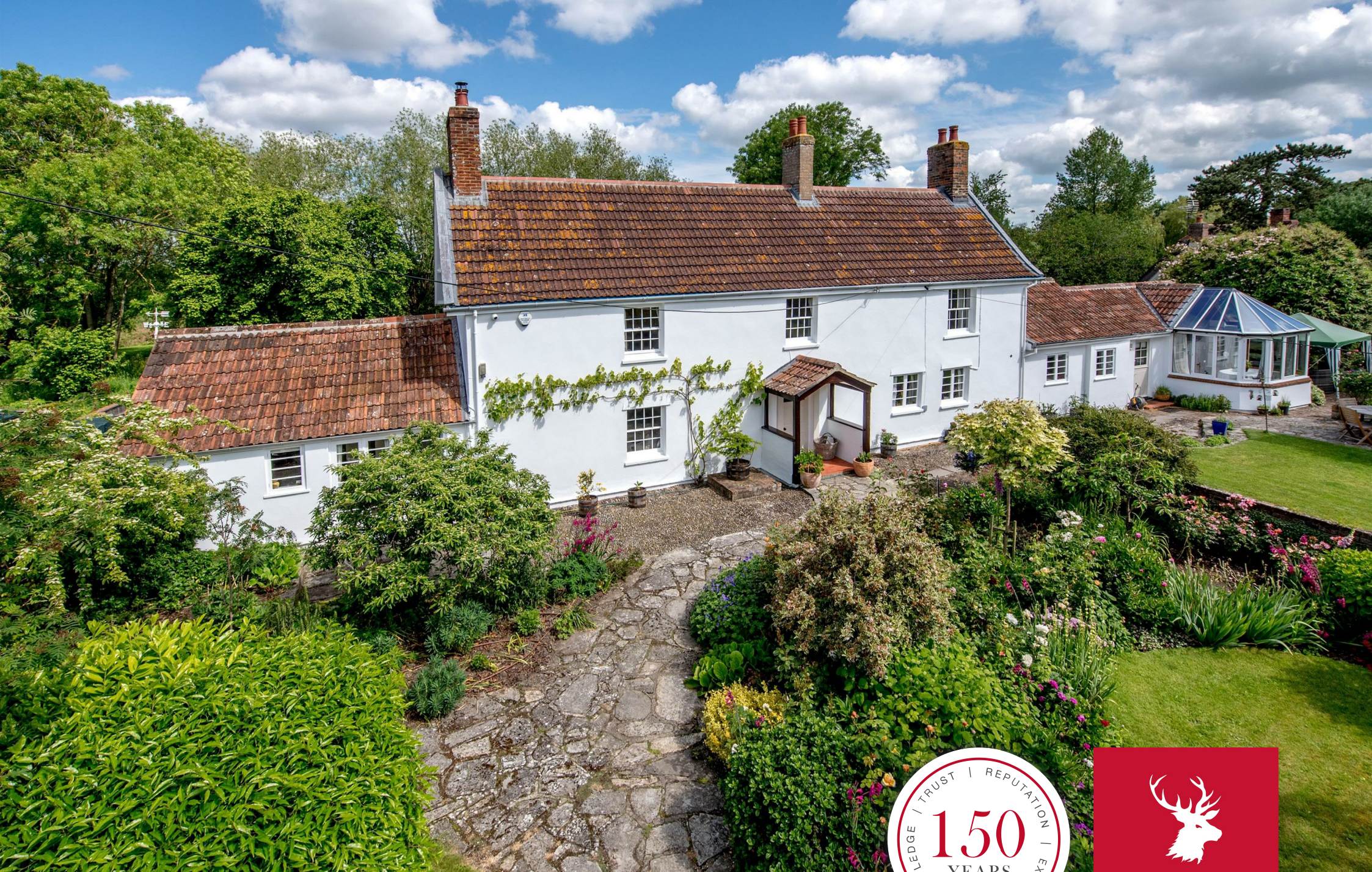
Ham Wharf House
