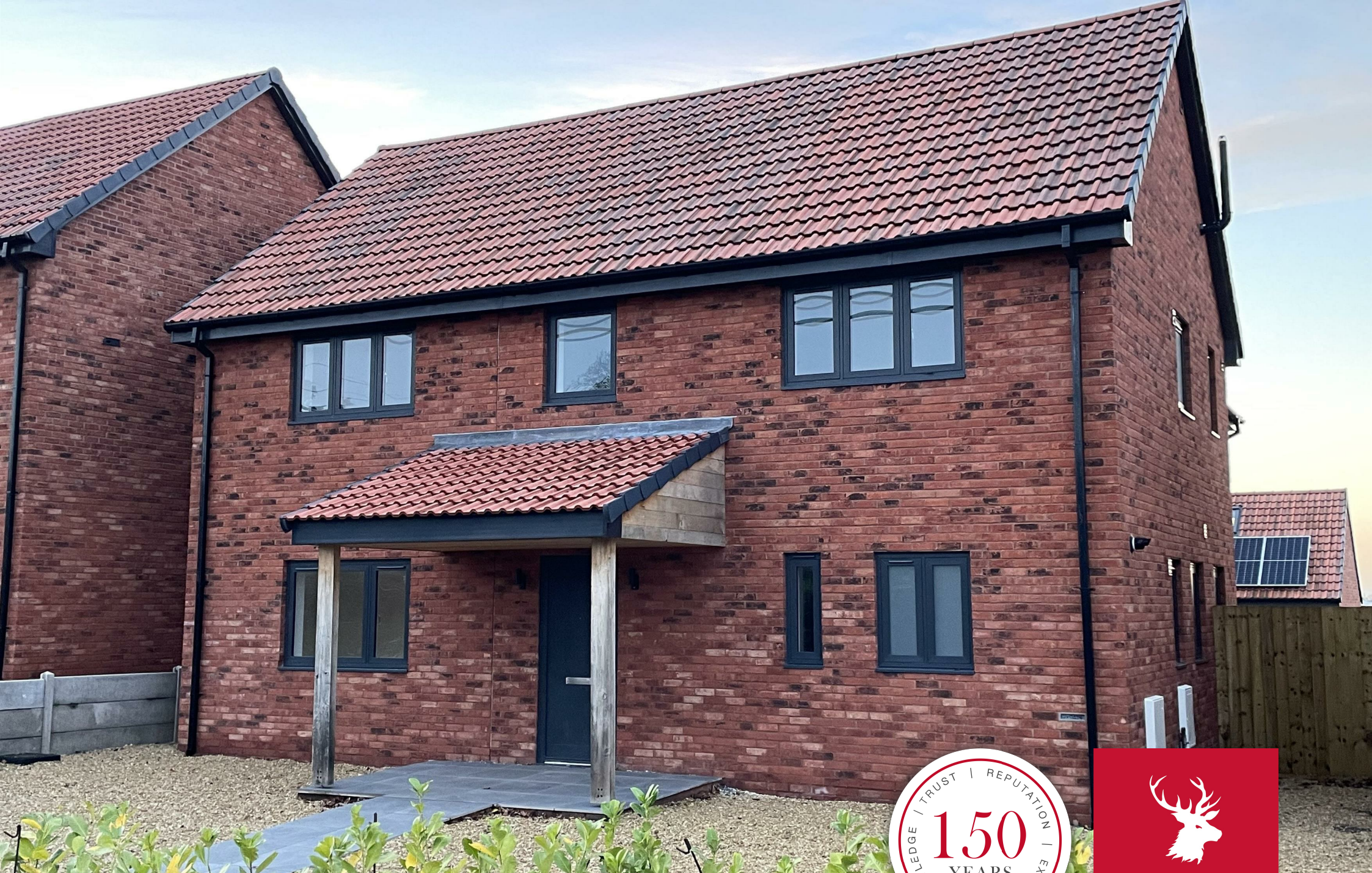
Edgar House, North Lane
