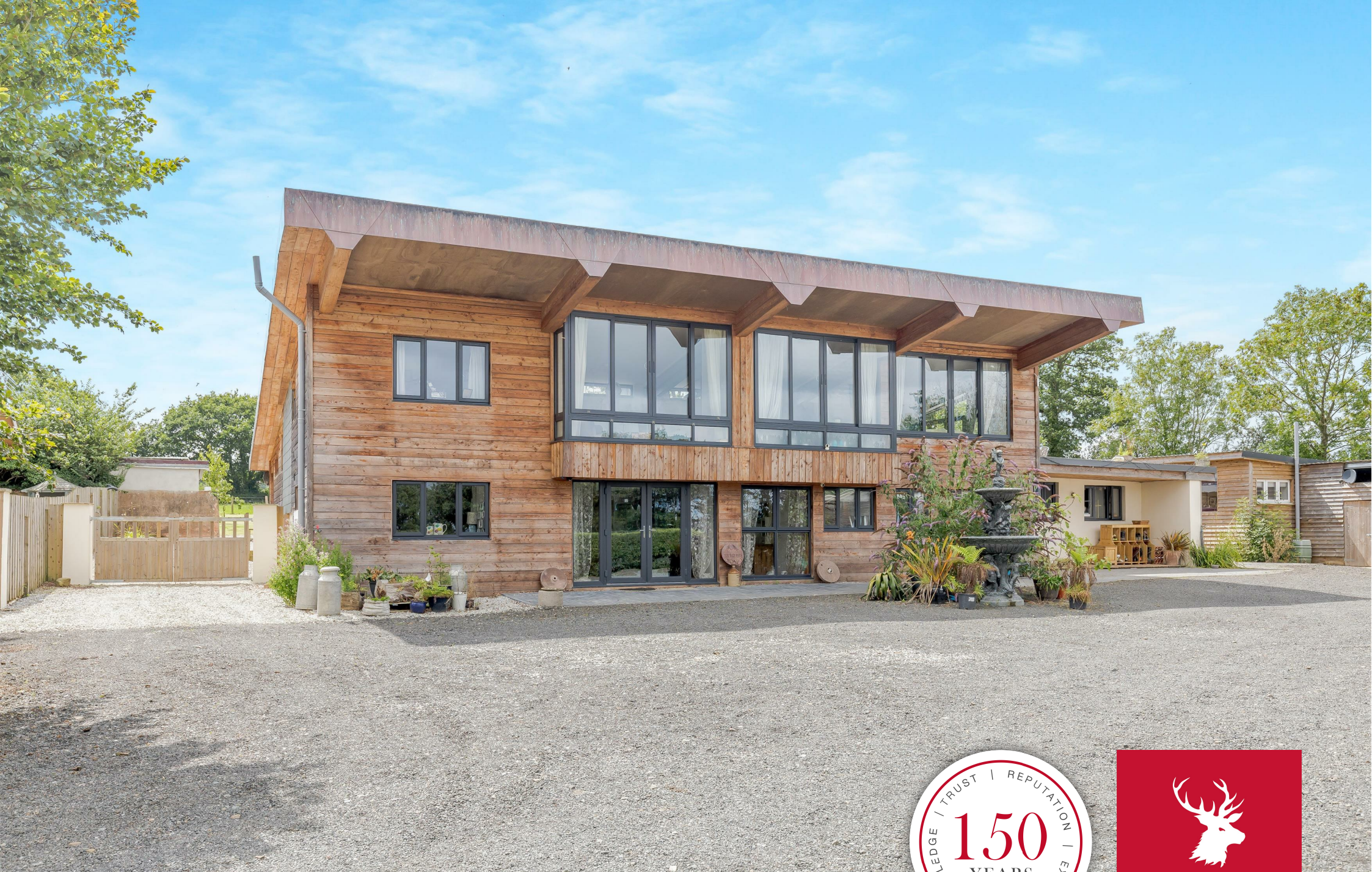
Tor Yard Barn
