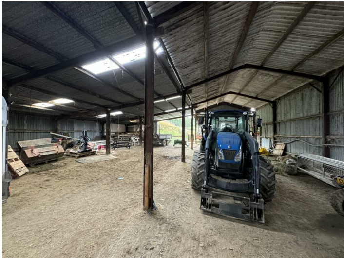
of steel framed construction being zinc clad with zinc roof over.
