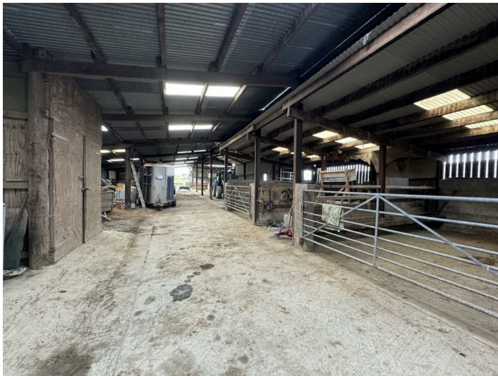
of steel framed construction being zinc clad with zinc roof over.
