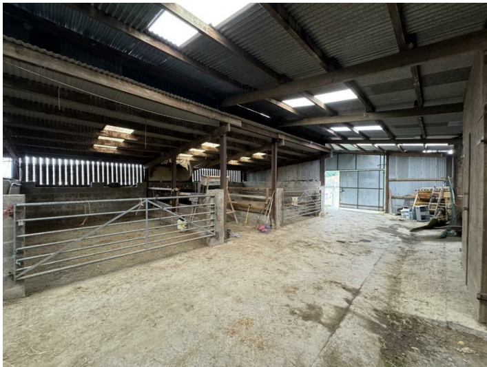
19' x 25' (5.79m x 7.62m ) of timer framed construction being zinc clad and open ended to front providing excellent dry storage area.
