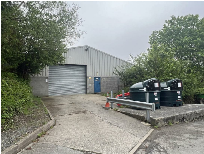
Currently utilised by the ground maintenance department. The layout is highlighted on the Rheidol building floor plan.
