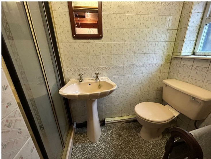
Shower cubicle, two piece suite, fully tiled walls.
