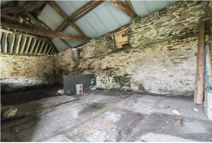
Internals of Barn One
