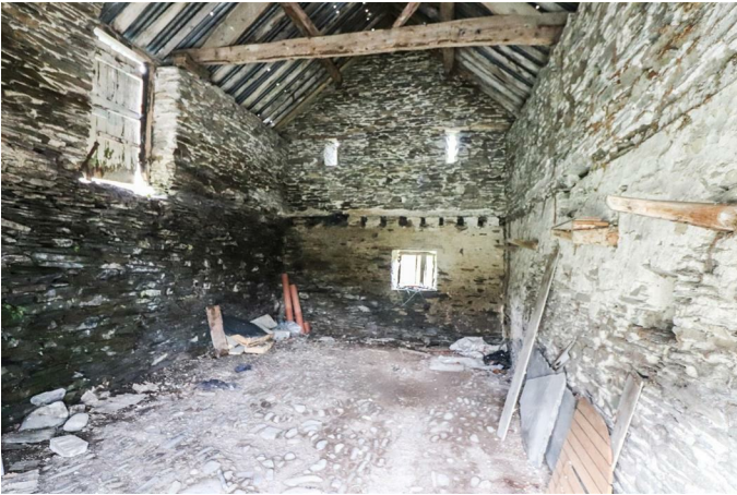
Internals of Barn Two
