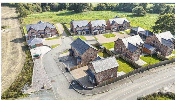
An Aerial View of the Development
