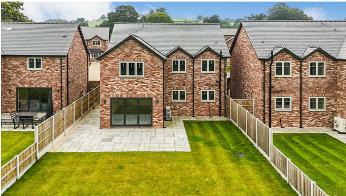
To The Rear Of The Property
