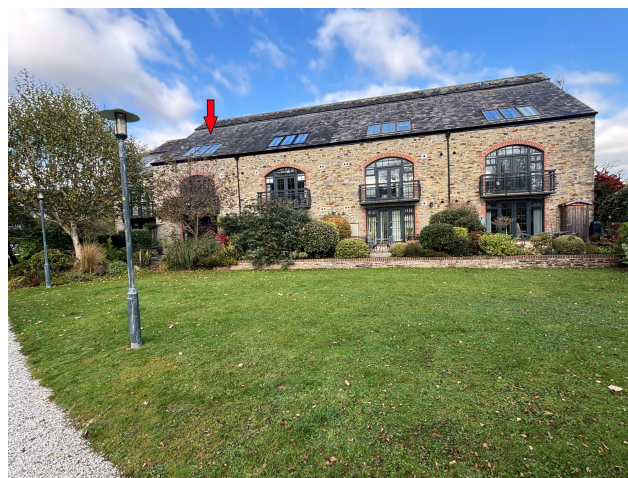
REAR ELEVATION OF THE BUILDING
