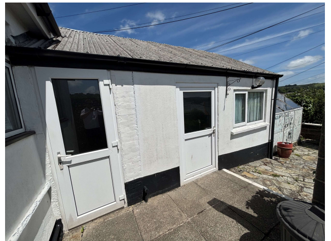
OUTSIDE W.C AND UTILITY ROOM/STORE
