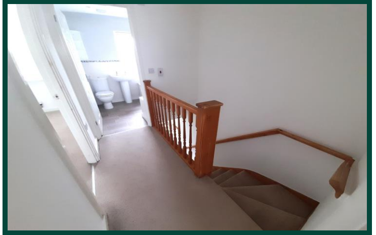
STAIRS AND LANDING
