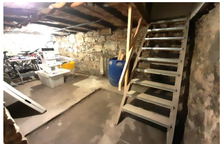
Cellar 1 - Storage and Stairs
