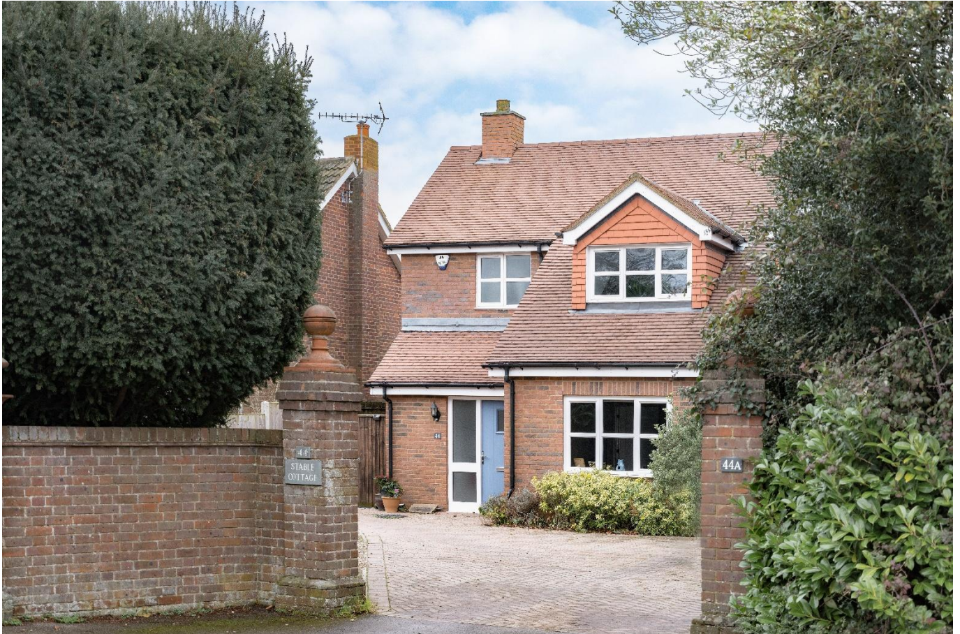
Stable Cottage, 44 Grove Road, Tring, Hertfordshire HP23 5PD
