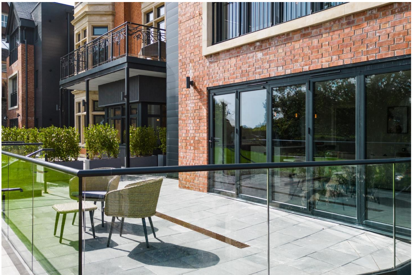
Apartment 1, Ashdene Manor, 10 Bridgeman Road, Penarth, The Vale Of Glamorgan, CF64 3AB
