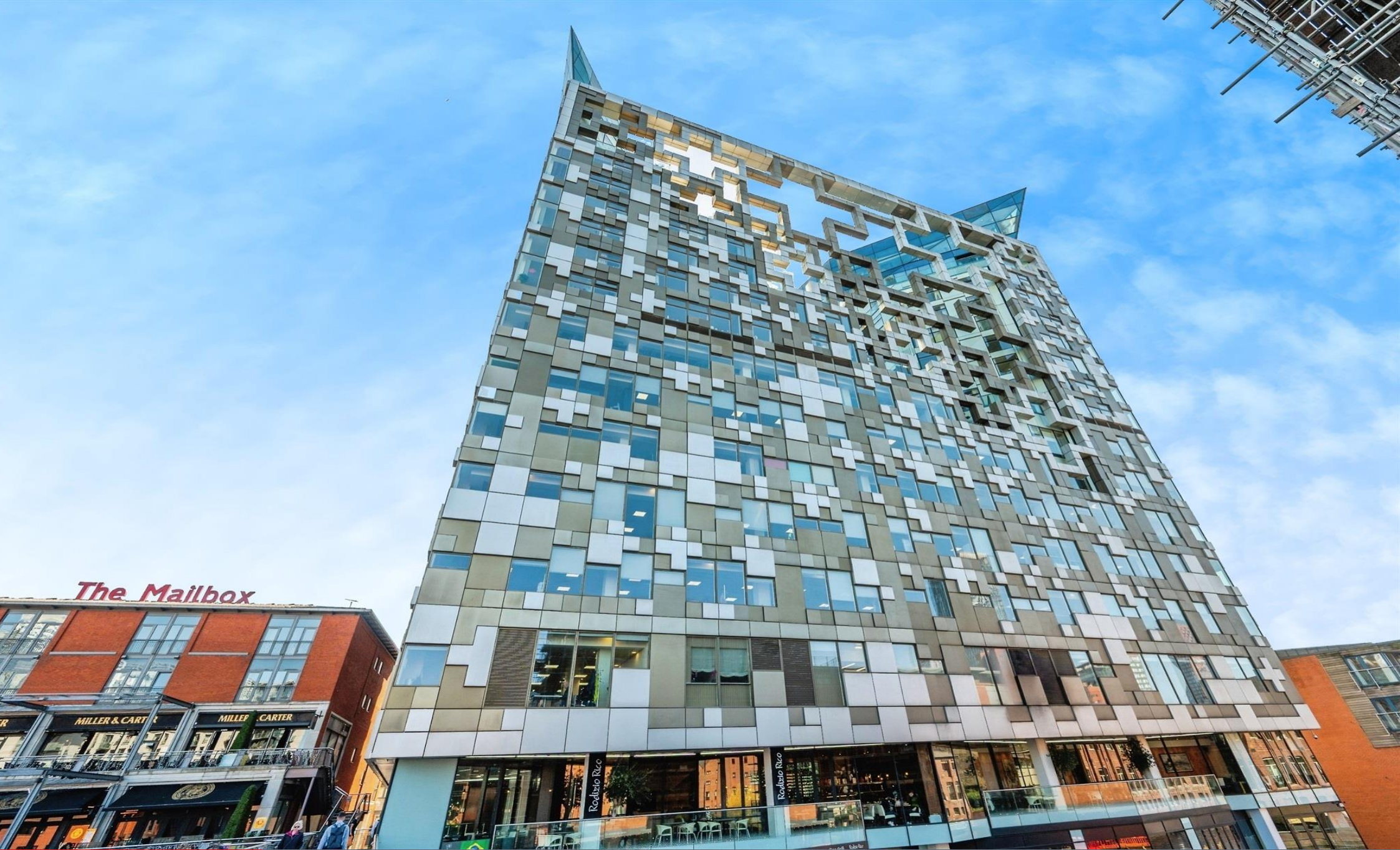
The Cube East Wharfside Street Birmingham
