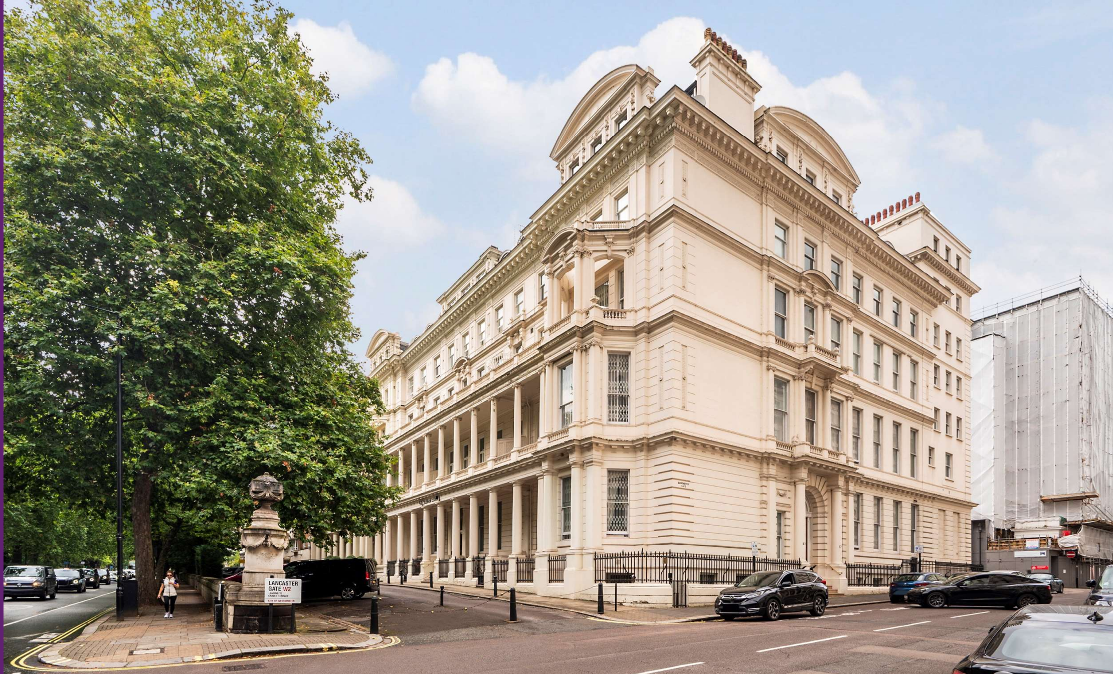
Blenheim Court Lancaster Gate, W2
