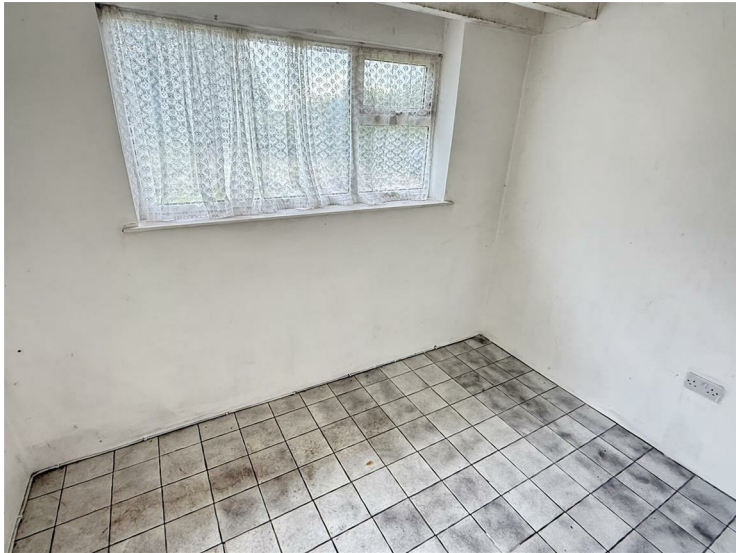
Side Porch/Utility Room
