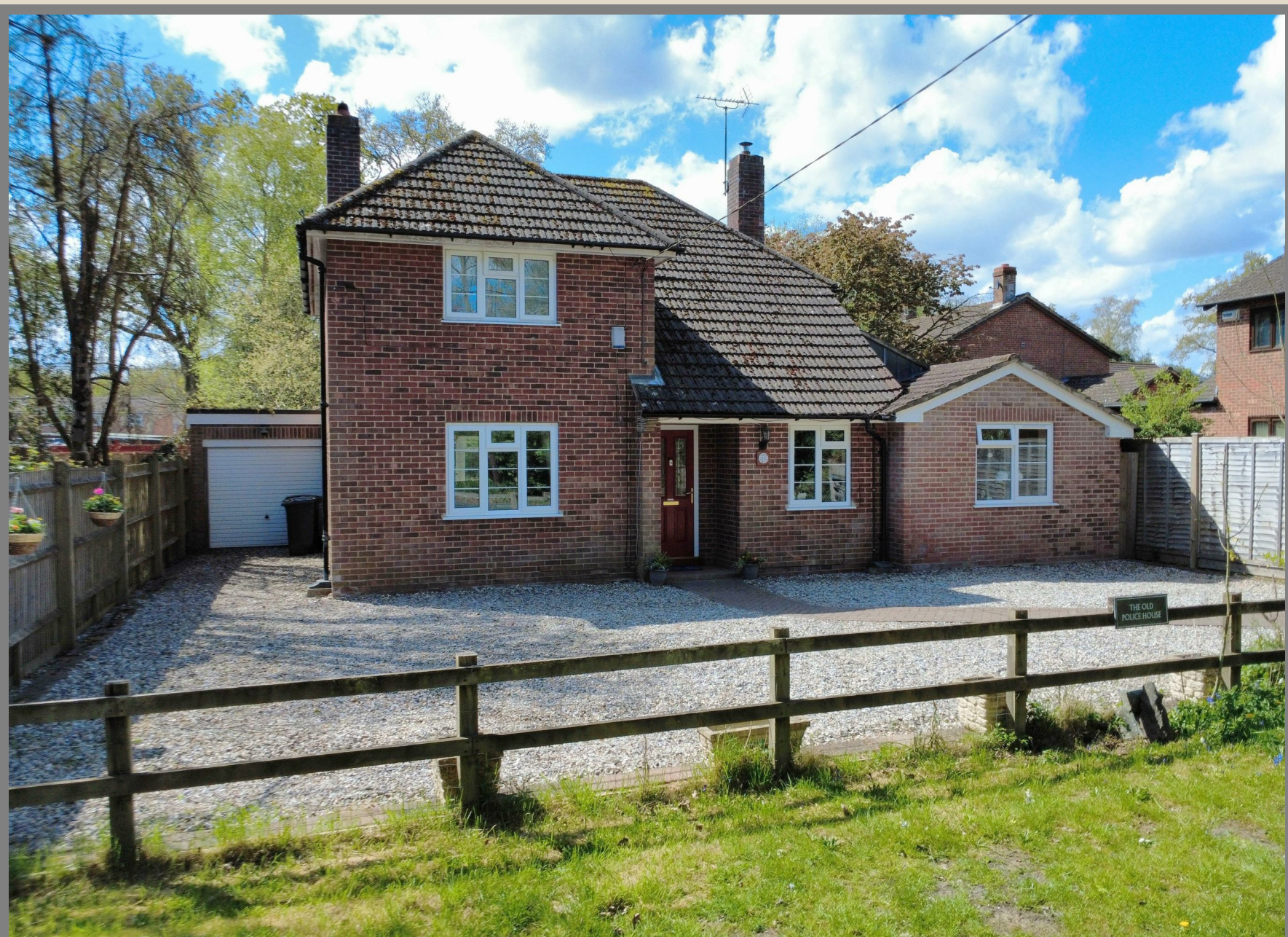
The Old Police Station, Penwood, Highclere, RG20 9EX
