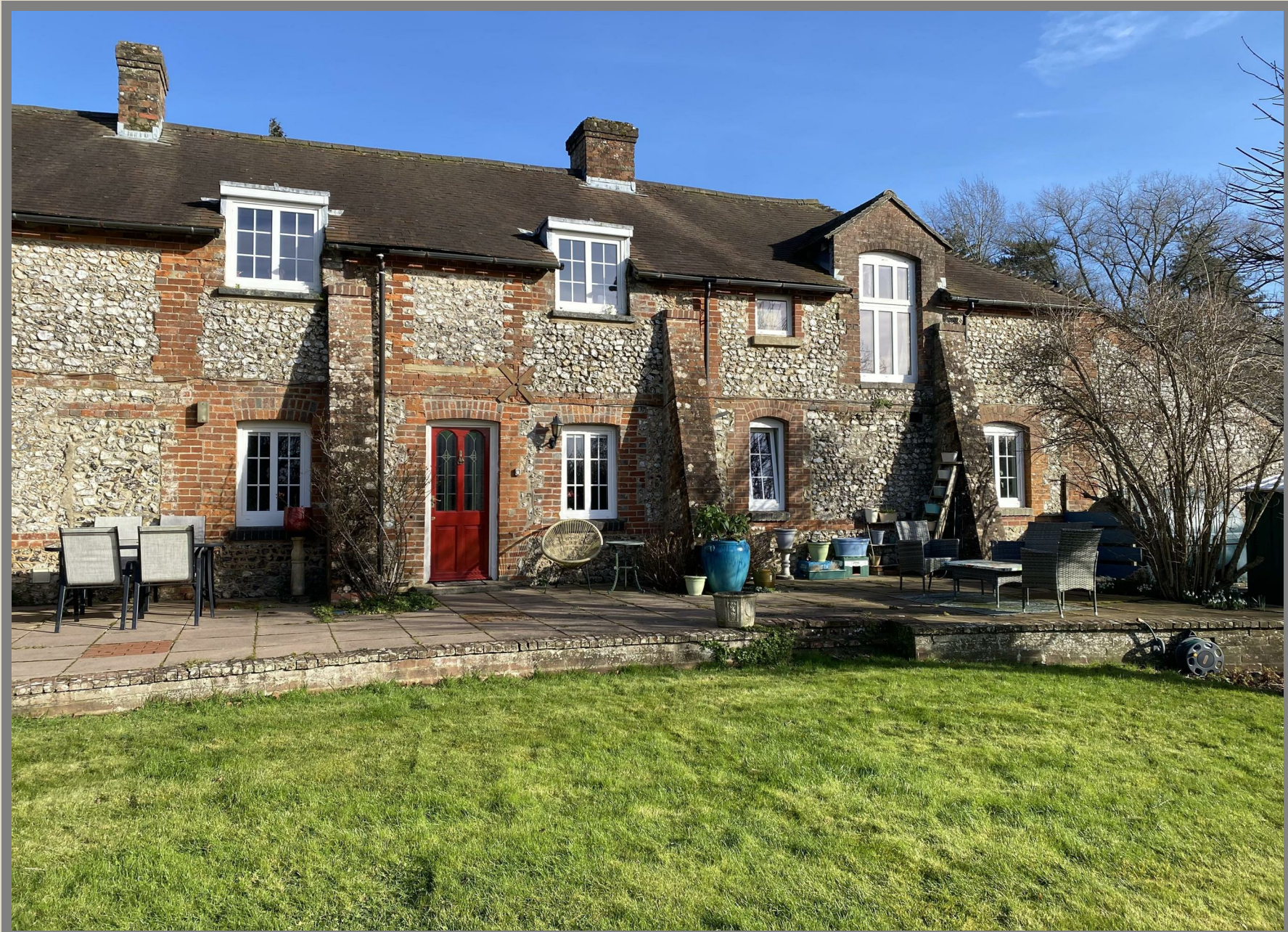
Stable Cottage, Esseborne Manor, Hurstbourne Tarrant, Andover, SP11 0ER
