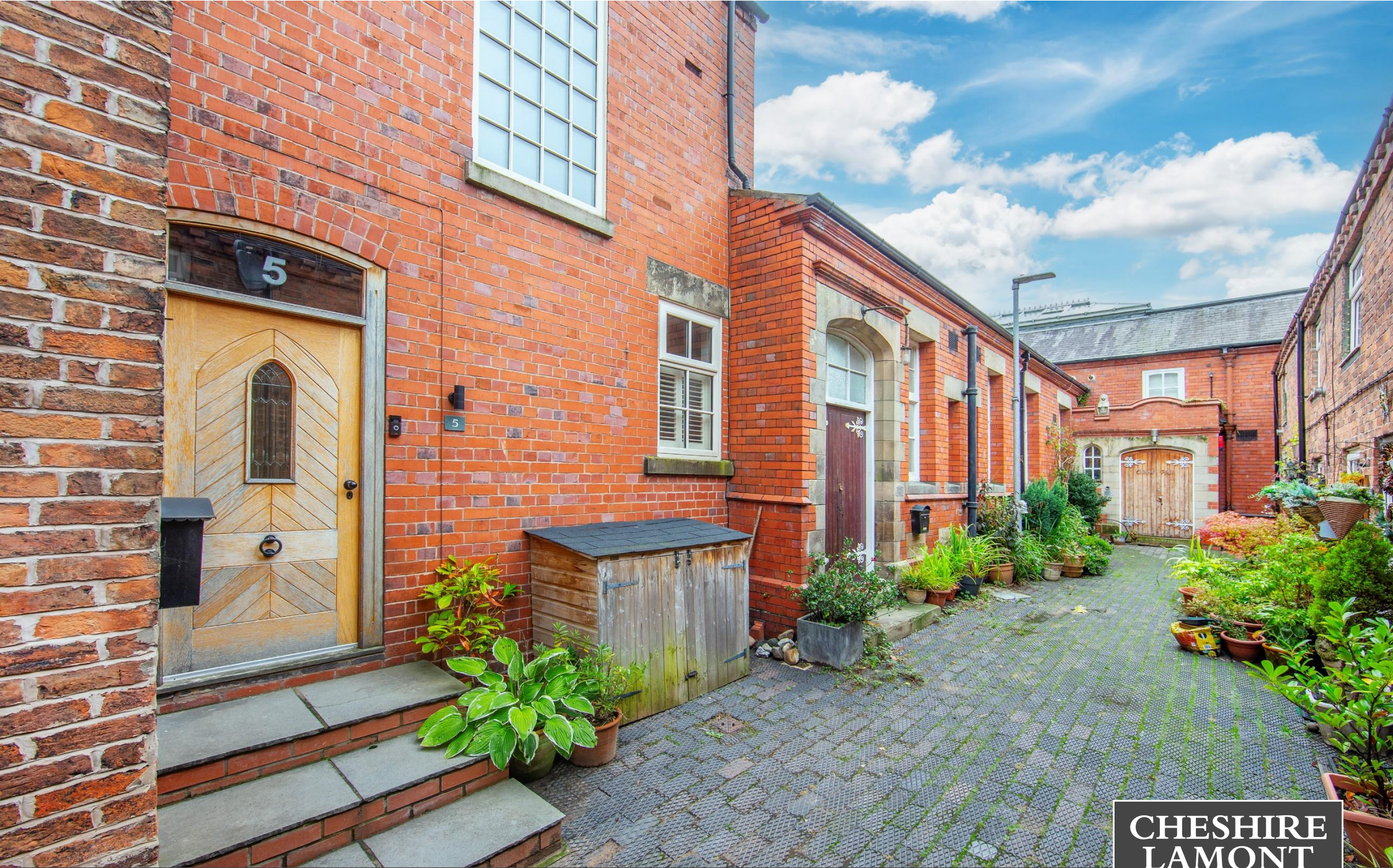
“Chapel House”, 5 Chapel Row, Nantwich CW5 5EX
