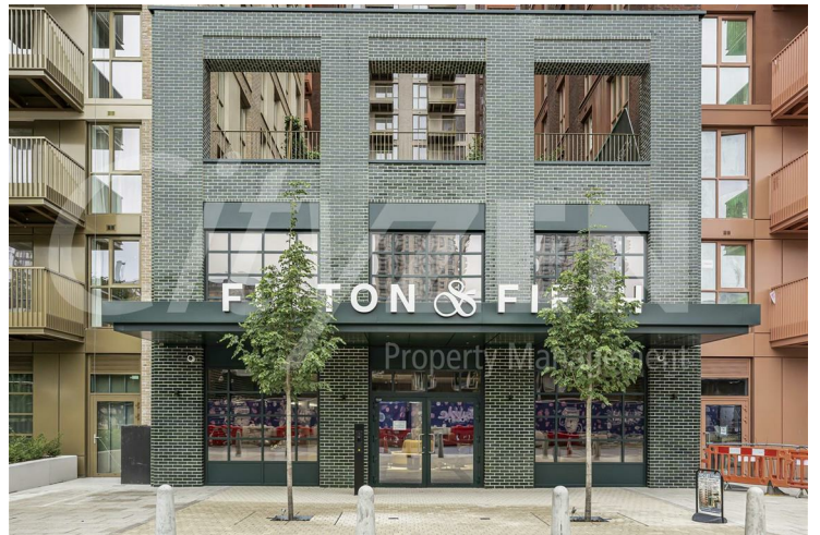
FULTON AND FIFTH ROOF GARDEN
