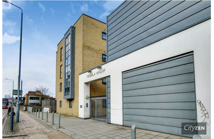
TEQUILA WHARF DEVELOPMENT
