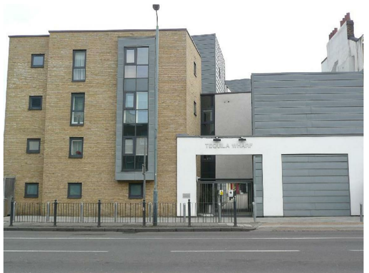
TEQUILA WHARF ENTRANCE
