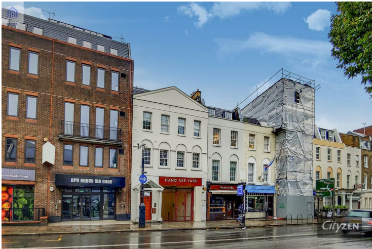
ACCESS FROM GRAY'S INN ROAD
