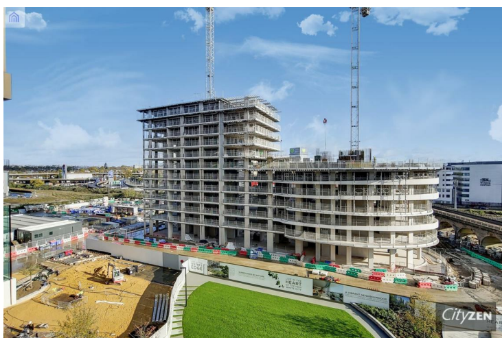
SOUTHERLY VIEW FROM BALCONY
