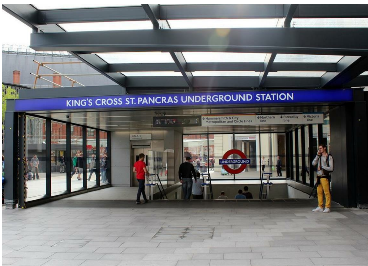
KINGS CROSS UNDERGROUND STATION
