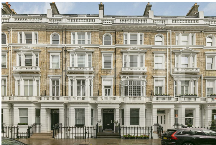
EXTERNAL OF BUILDING
