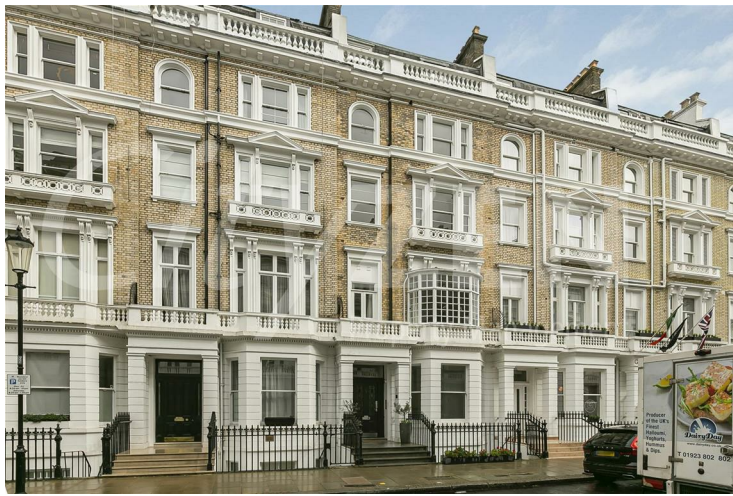
EXTERNAL OF BUILDING
