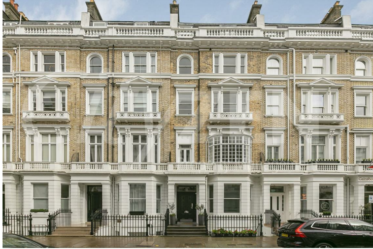
EXTERNAL OF BUILDING
