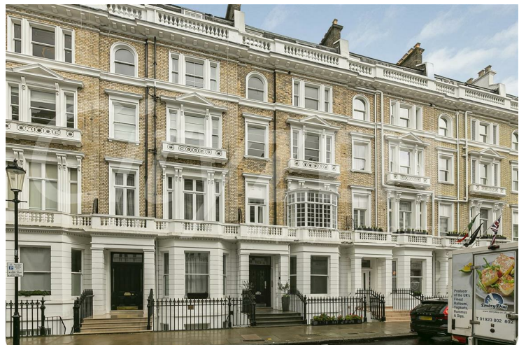
EXTERNAL OF BUILDING
