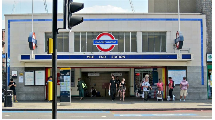
MILE END STATION
