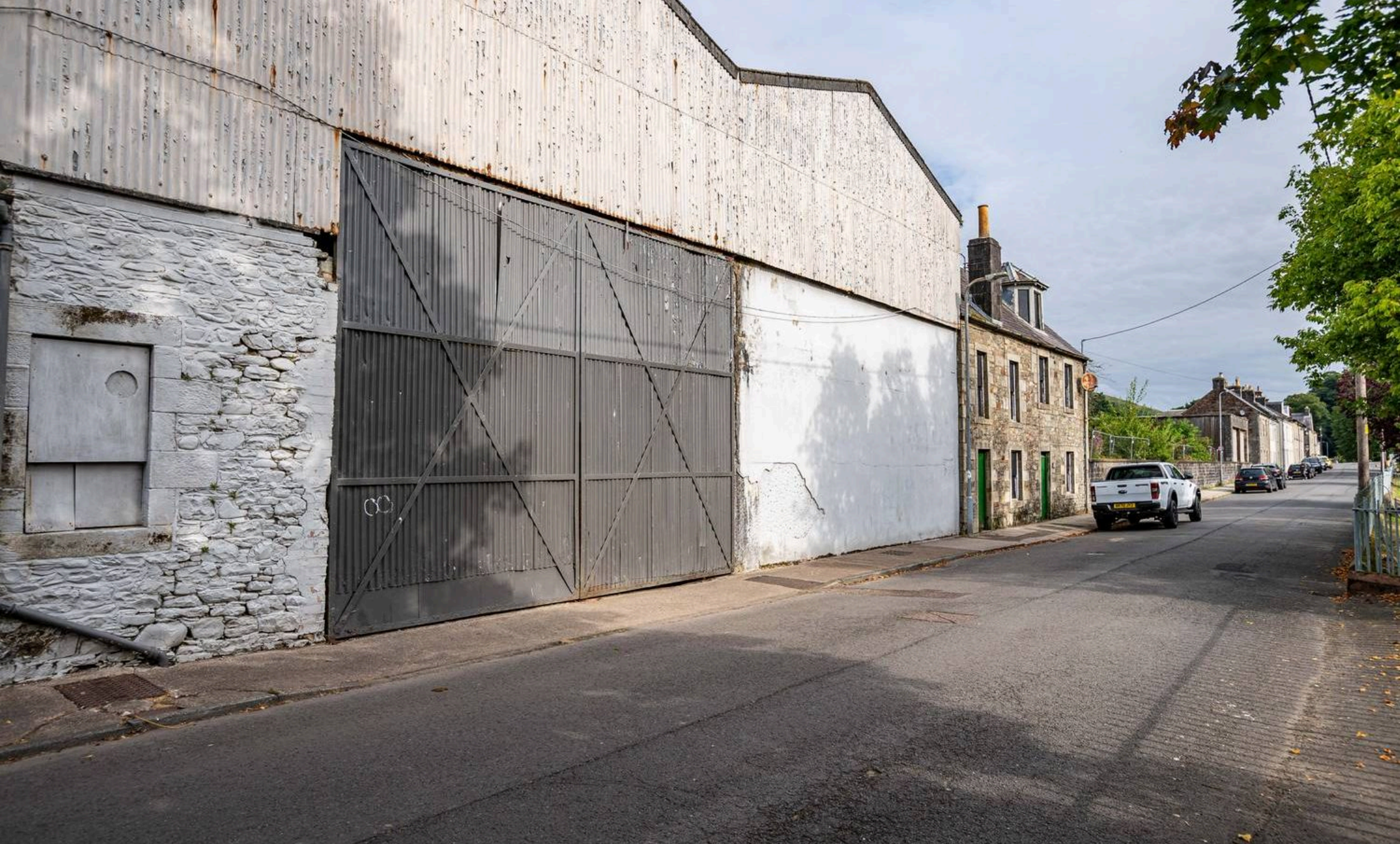
Storage Unit, Elizabeth Street, Langholm, DG13 0AJ £400 pcm
