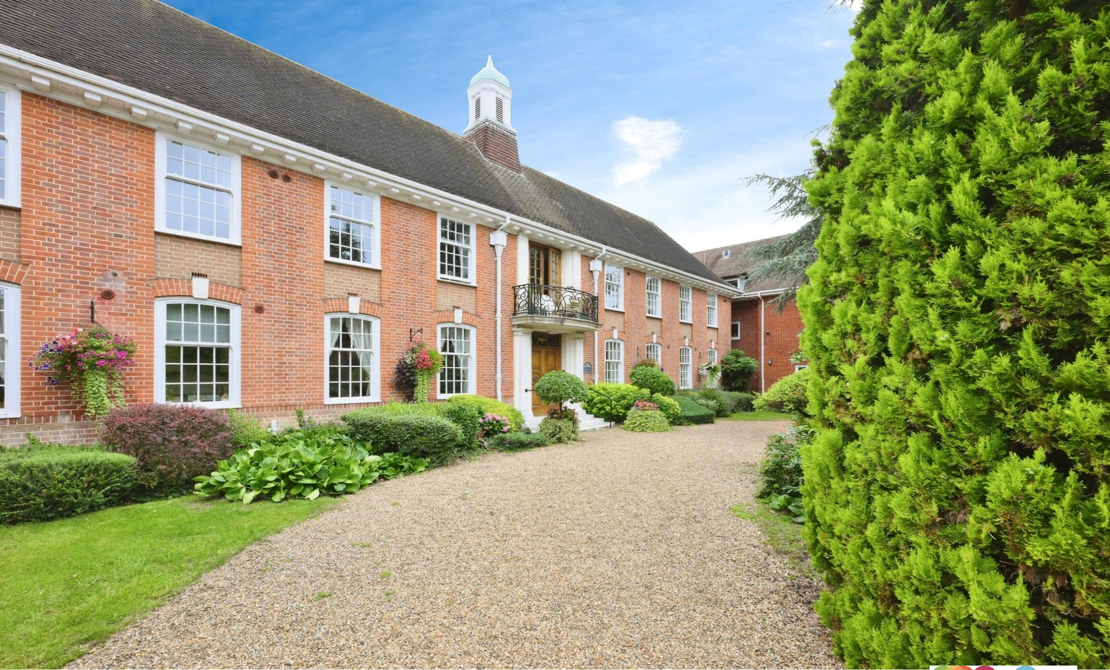
Belvedere Court High Street, Hoddesdon EN11 8UX
