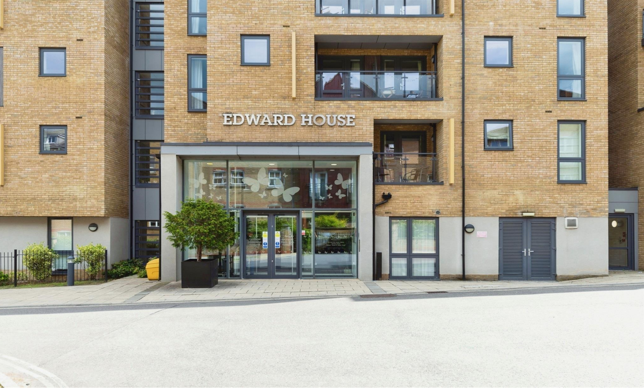
Edward House Pegs Lane, Hertford, SG13 8FQ
