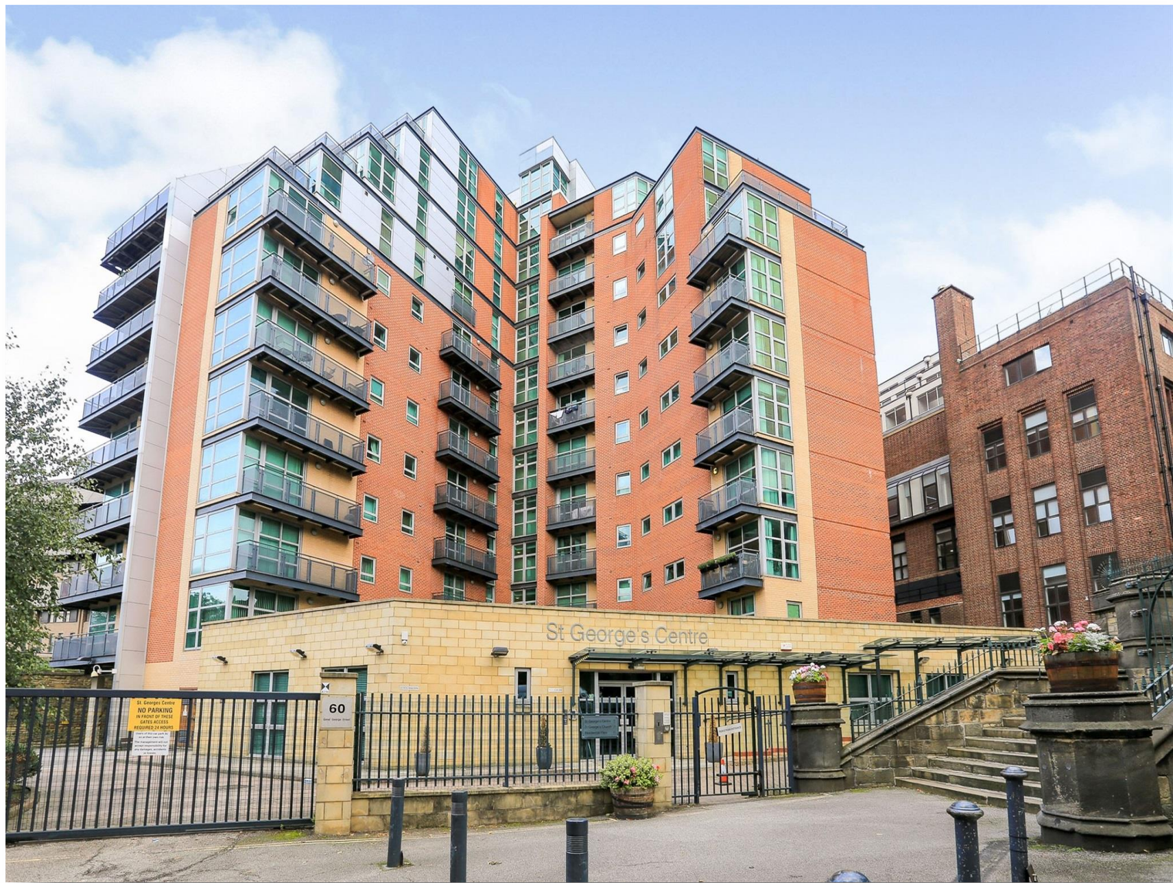
The St George Building Great George Street, City Centre Leeds LS1 3DL
