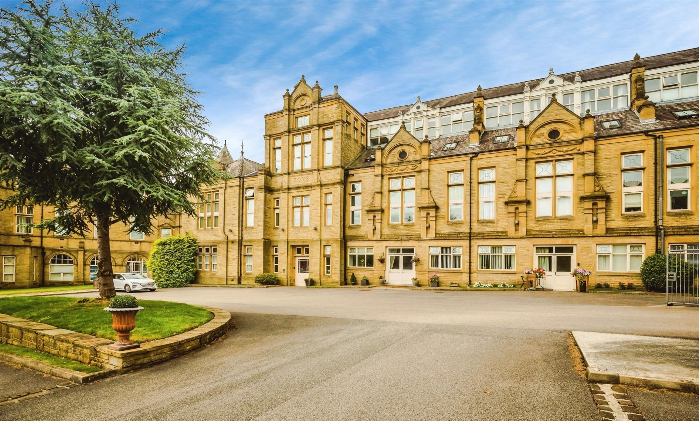
Clare Hall Apartments Prescott Street, Halifax HX1 2HQ
