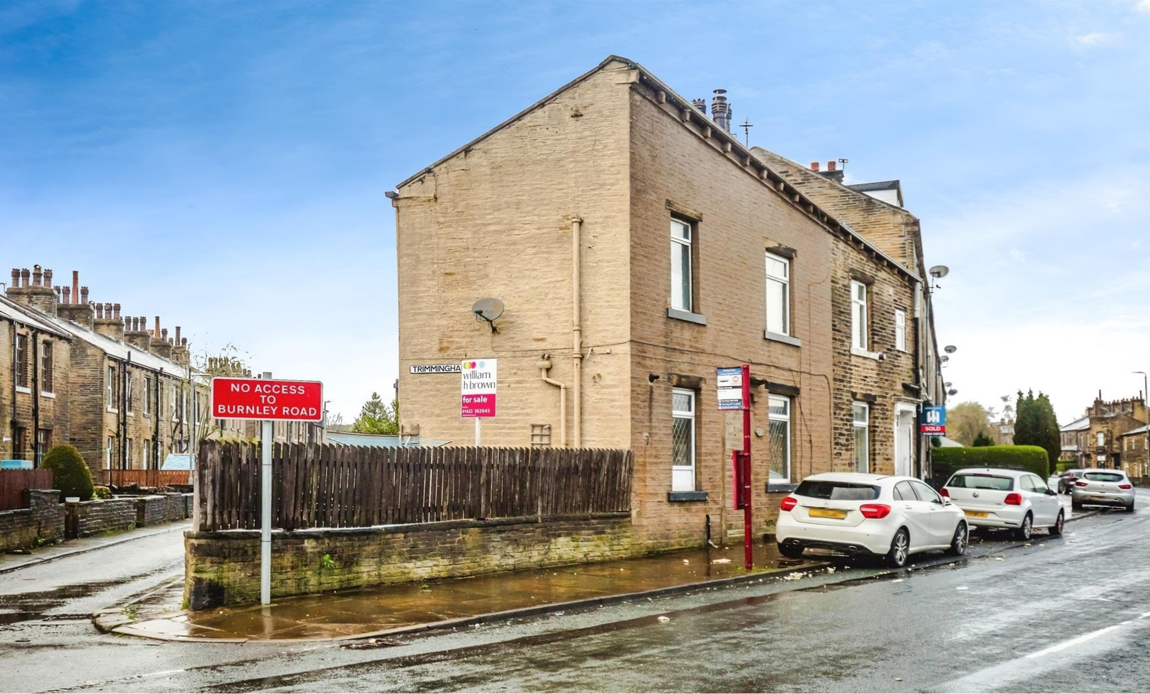
Warley Road, HALIFAX HX1 3TW
