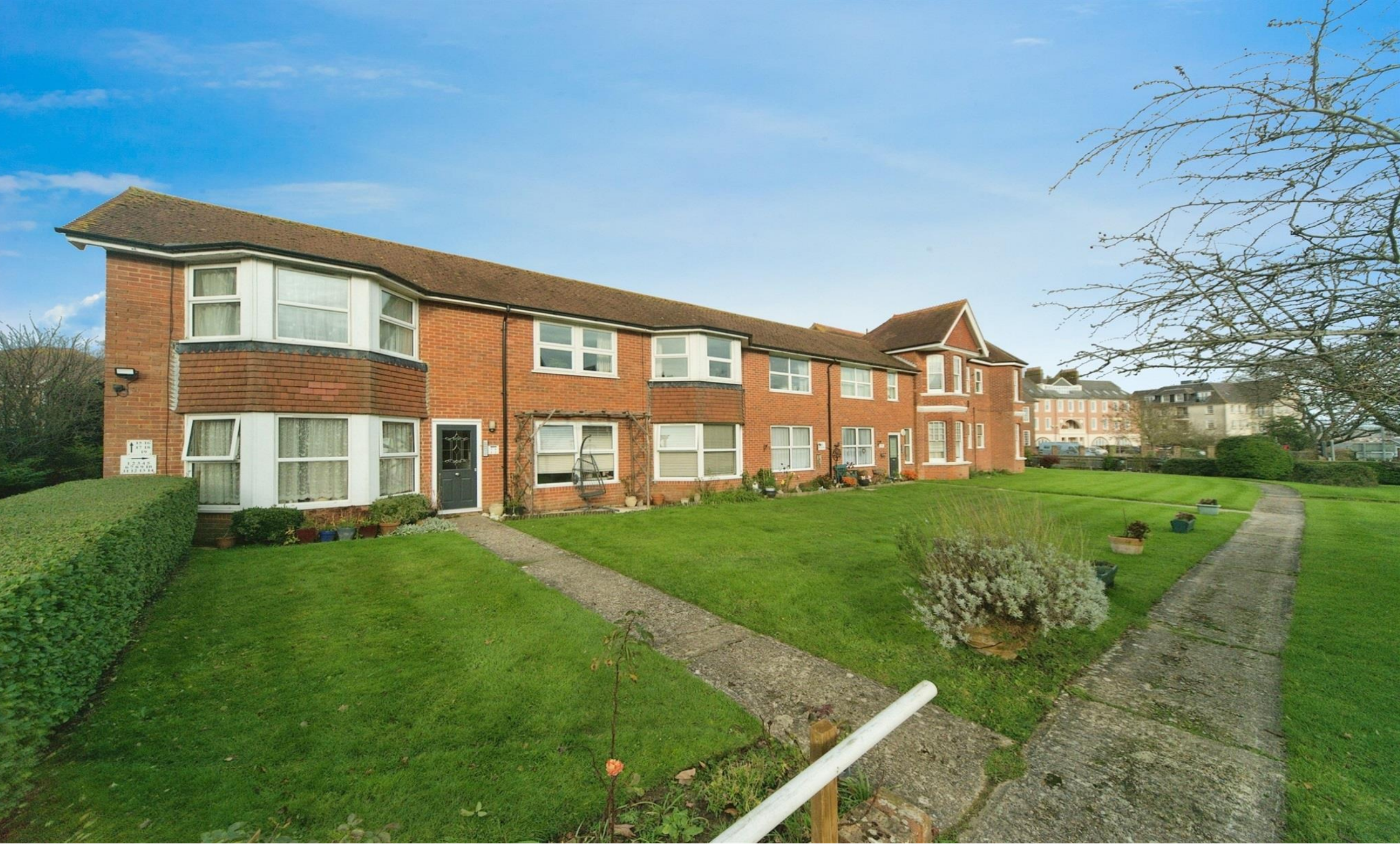
Laurel Bank Hastings Road, Bexhill-On-Sea TN40 2NH
