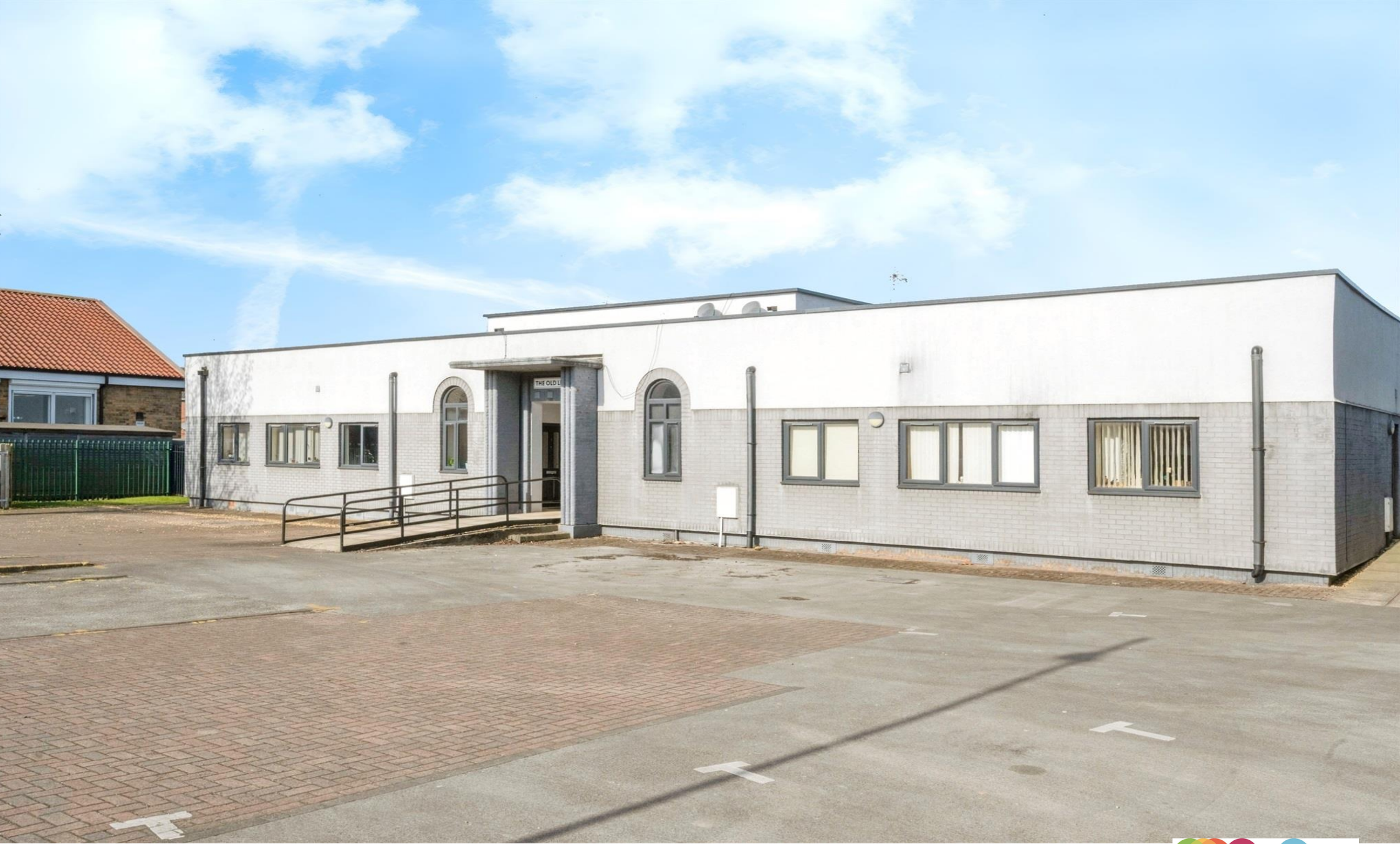
The Old Library Mcconnel Crescent, New Rossington Doncaster
