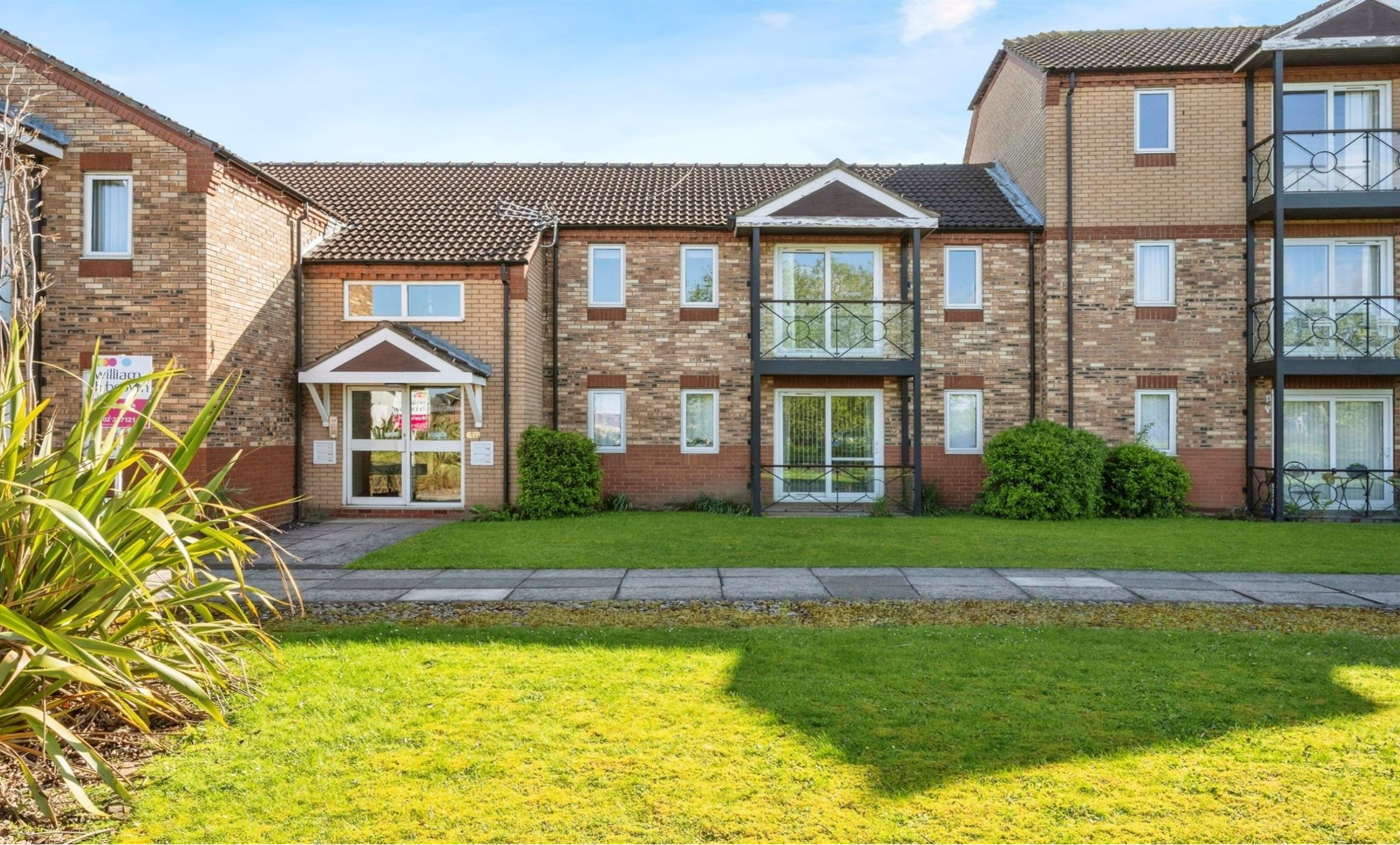
Lakeside Boulevard, Lakeside Doncaster
